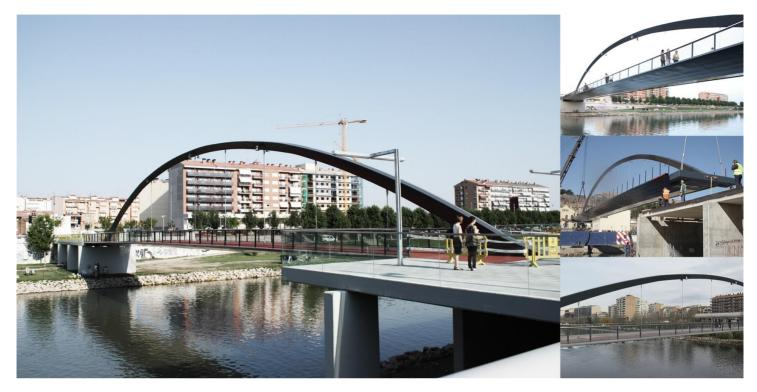
The Project has two different but perfectly integrated areas: firstly the accesses which constitute the link between the two pedestrian paths which run along the banks of the river, with the footbridge itself and the central span which corresponds to the flow of the River Segre, which is solved with an arch with lower deck construction.
